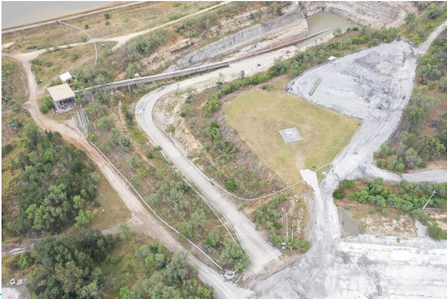
Underground Conveyor Infrastructure & Helipad
