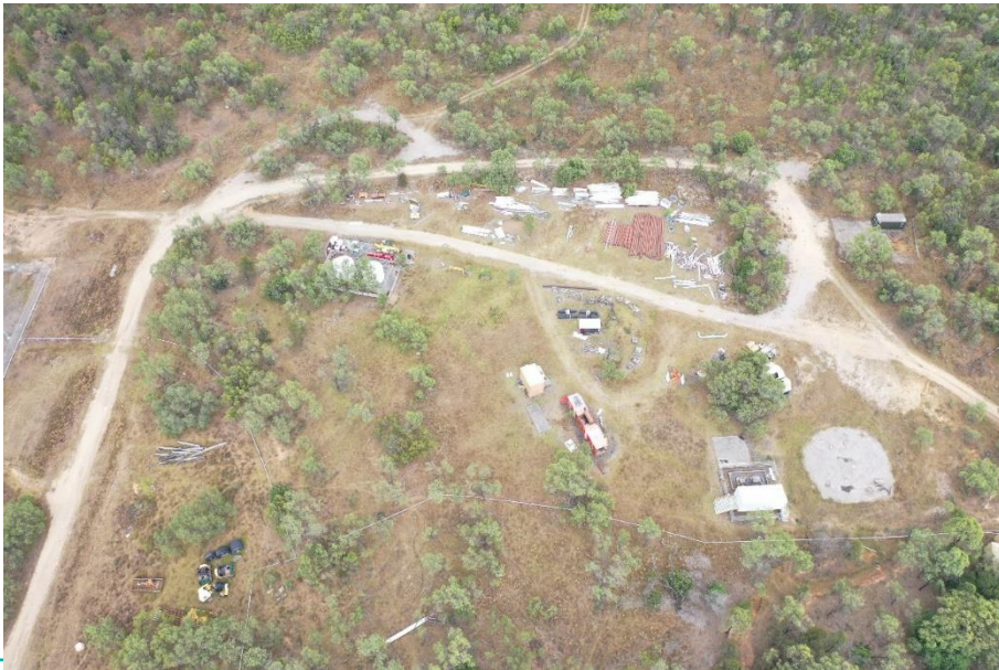
Western Hardstand Laydown
