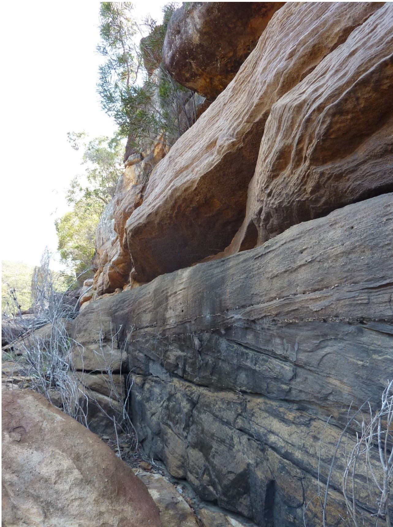
Photo C13-04 South End Looking Downstream
