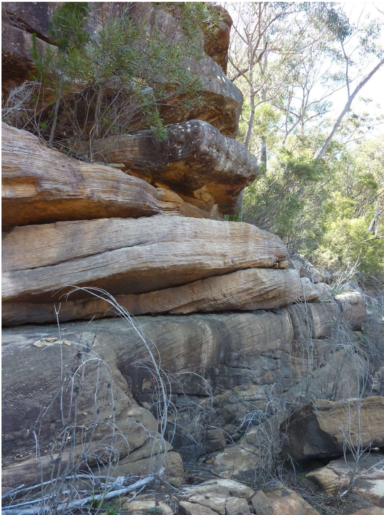
Photo C13-05 North End Looking Upstream
