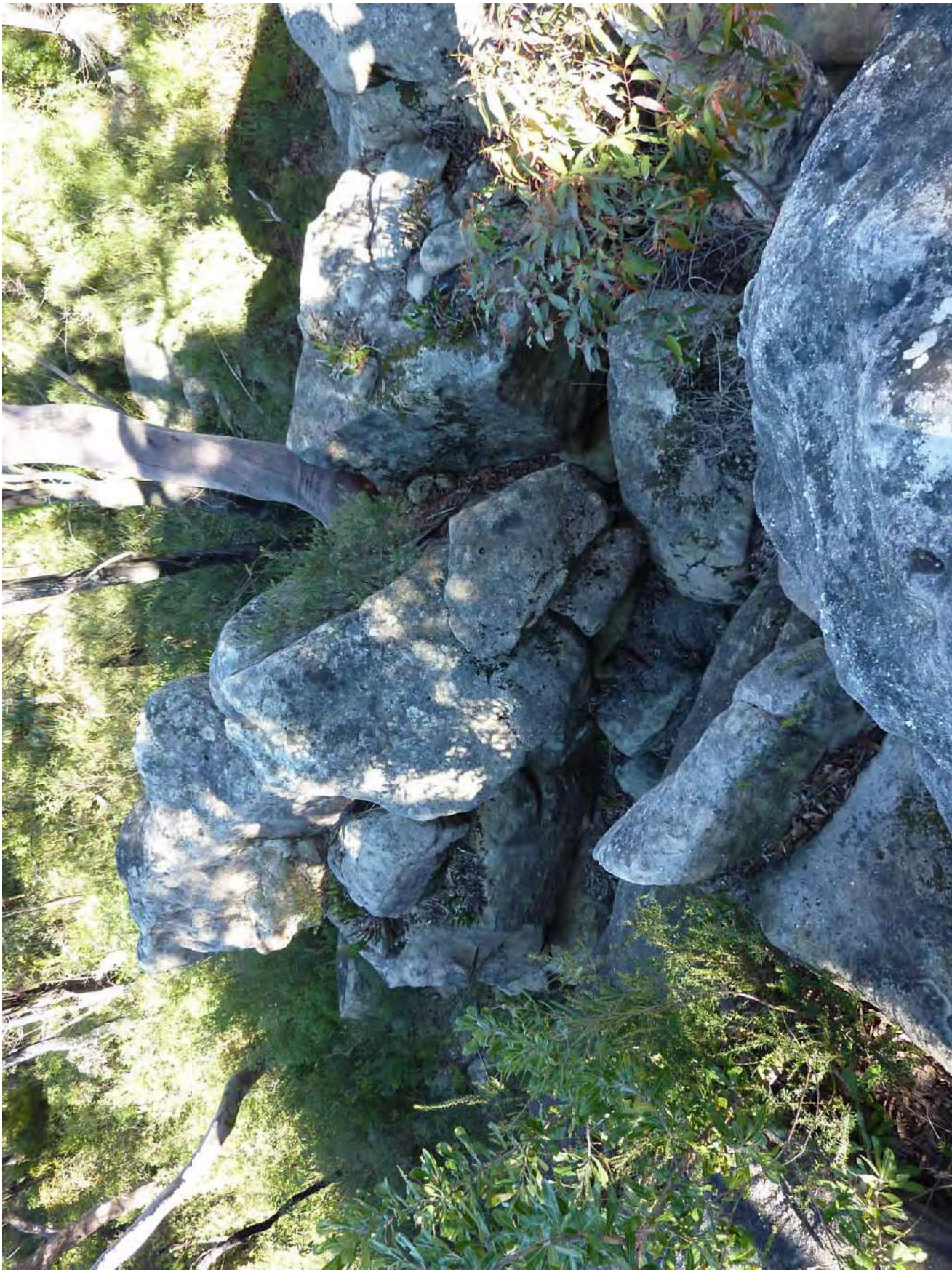
Photo C14-04 Detached blocks at western end of COH14
