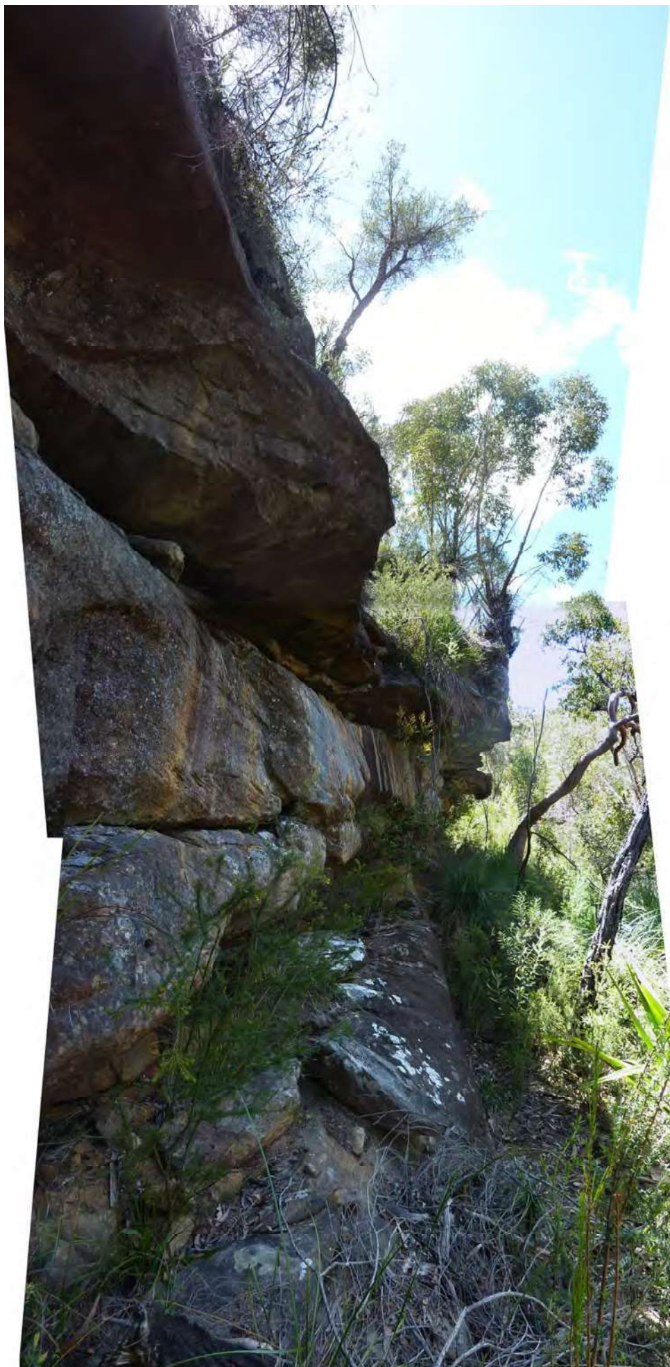
Photo C2-11 Rock ledge between overhangs, ~7.5m high
