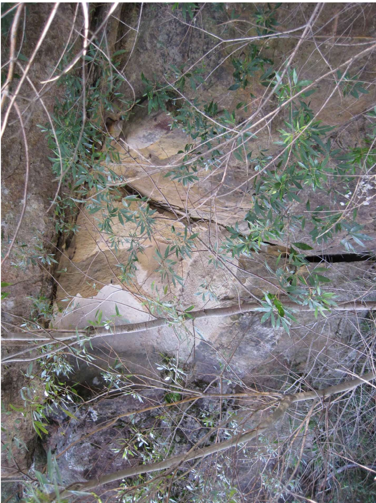
Photo C15-03 Eastern End – Existing Fracture in Rock
