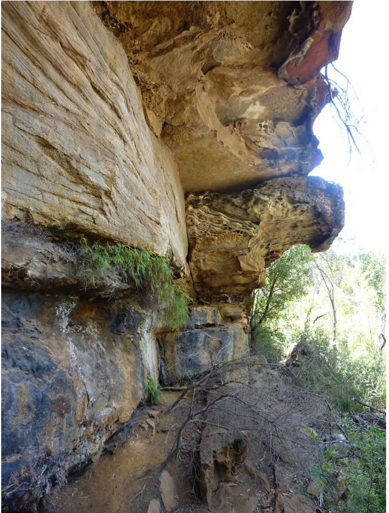
Photo C2-09 Looking north, overhang height ~6m, depth ~3m
