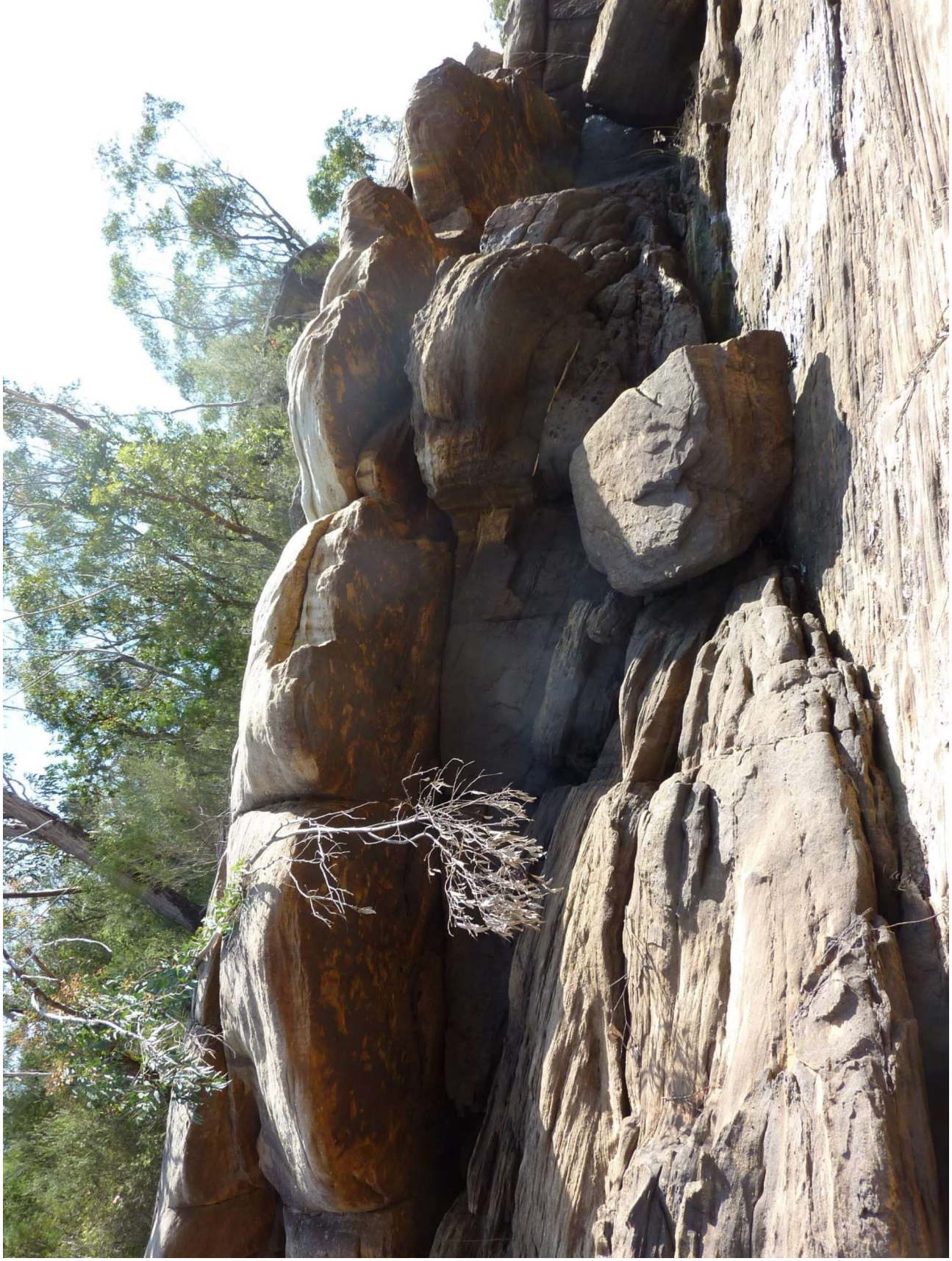
Photo C12-04 View Looking Upstream
