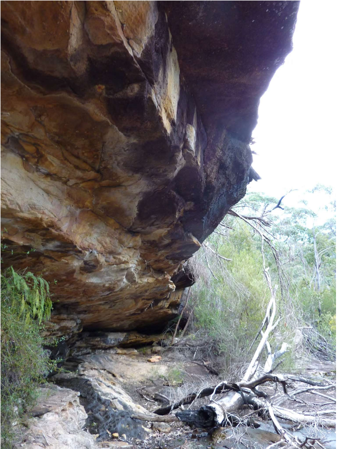
Photo C16-04 Overhang Looking Upstream
