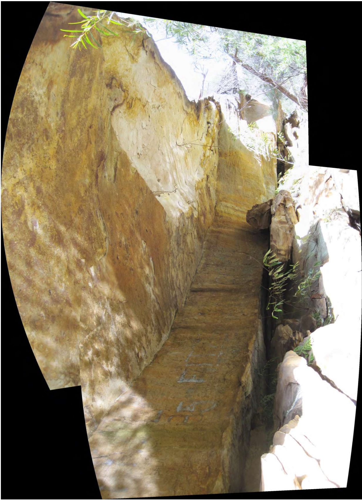
Photo C7-03 Eastern End Looking Upstream
