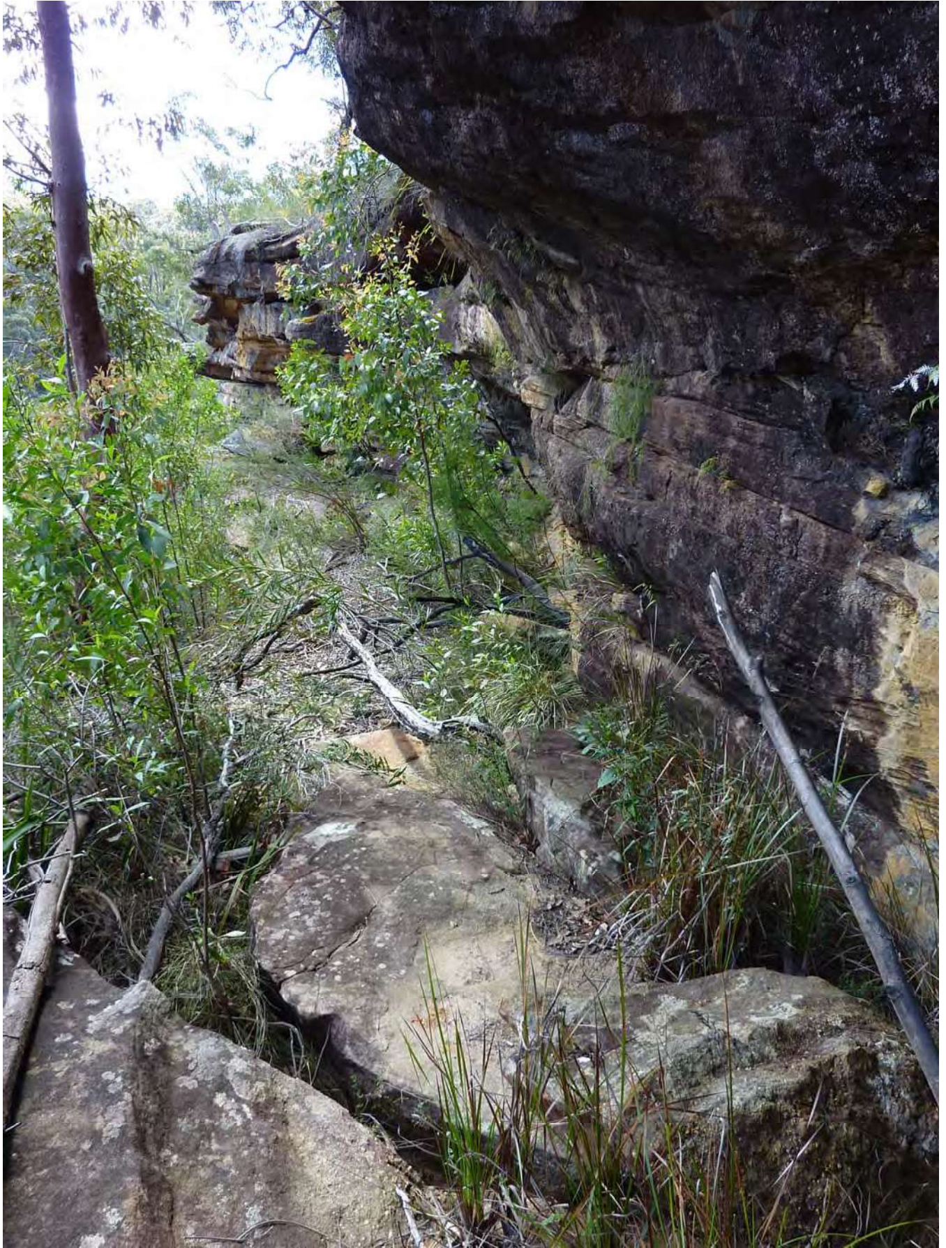
Photo C1-19 Large overhang looking north
