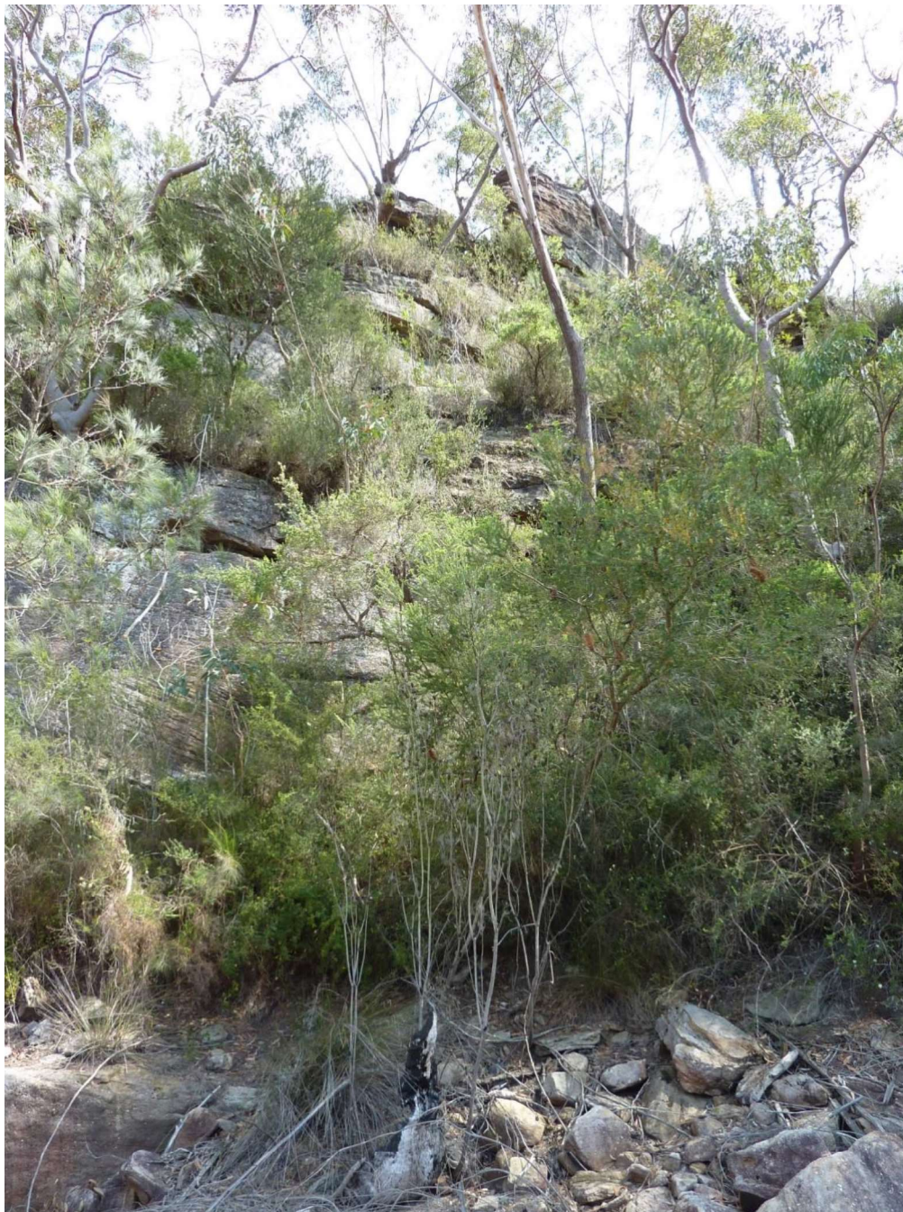
Photo C11-02 Eastern End Looking North West
